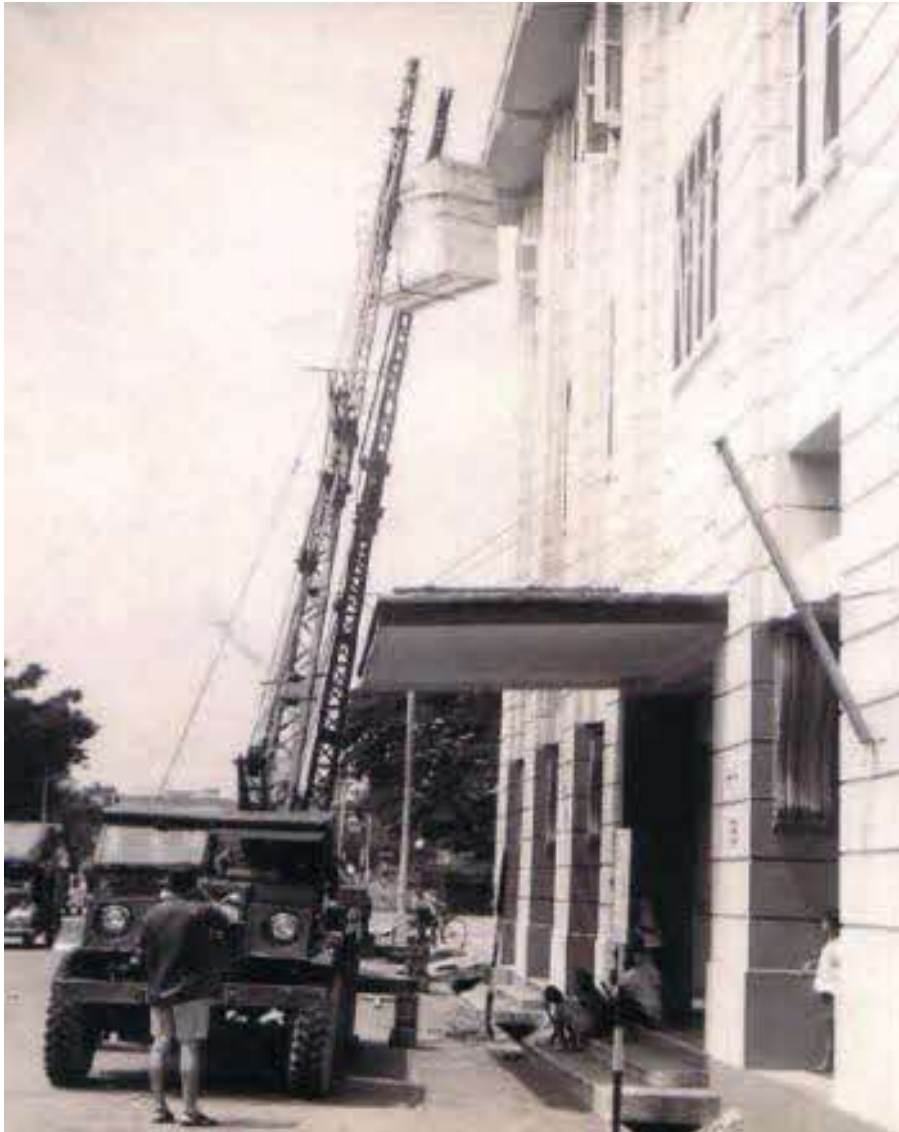
◀ Parts of the IBM1401 Data Processing System being lifted through the window at the CPF Board headquarters at 79 Anson Road. (Source: CPF Board)
